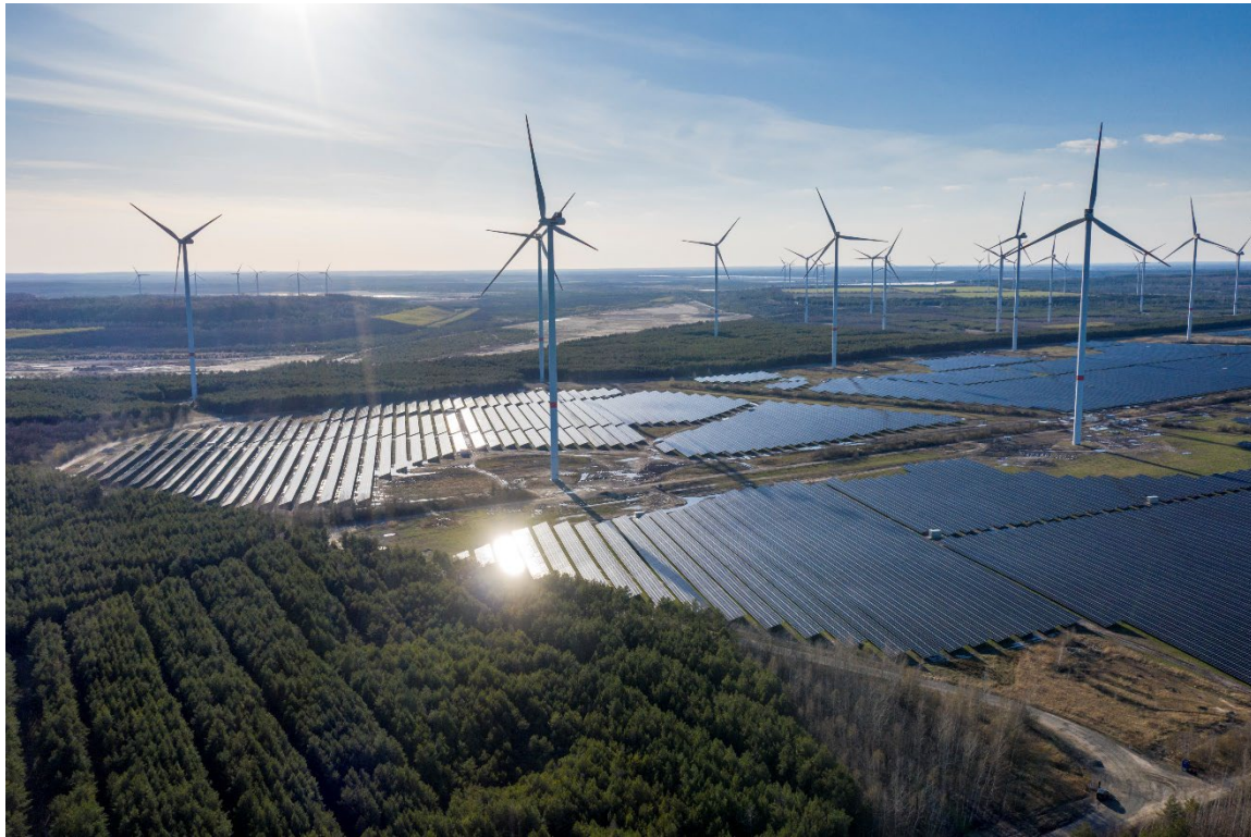
The first construction phase of the Lusatia Energy Park: Wind, PV and soon also hydrogen. (Photo: GP JOULE)
